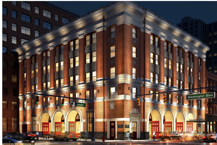
H1(a) Repurposed Historic Building
