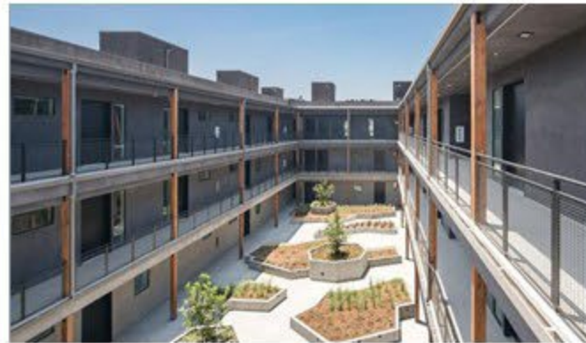
2980 Allesandro St. $3.62/SF Asking Rent 2017 Construction
