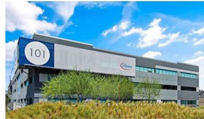
101 Pacific Coast Highway $51.60/SF Asking Rent 1987 Construction
