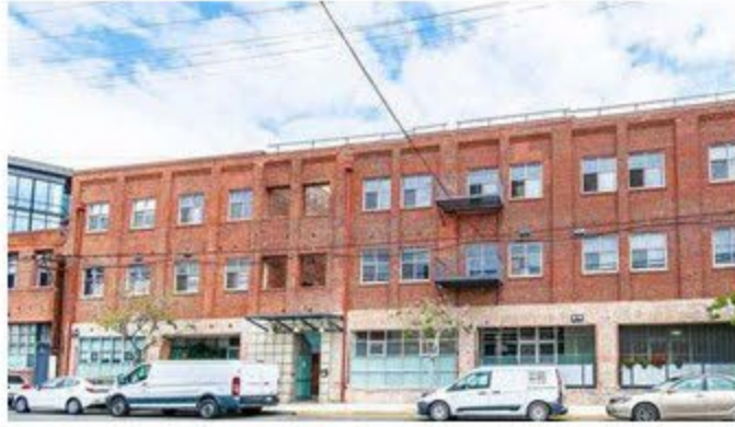
500 Molino St. $34.80/SF Asking Rent Industrial Adaptive Reuse
