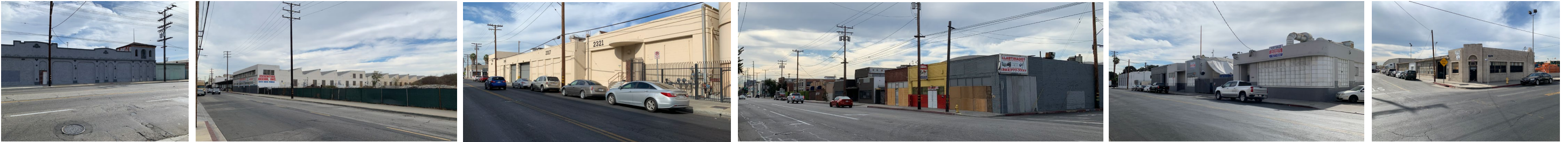
3 Active and Potential for Rehabilitation
