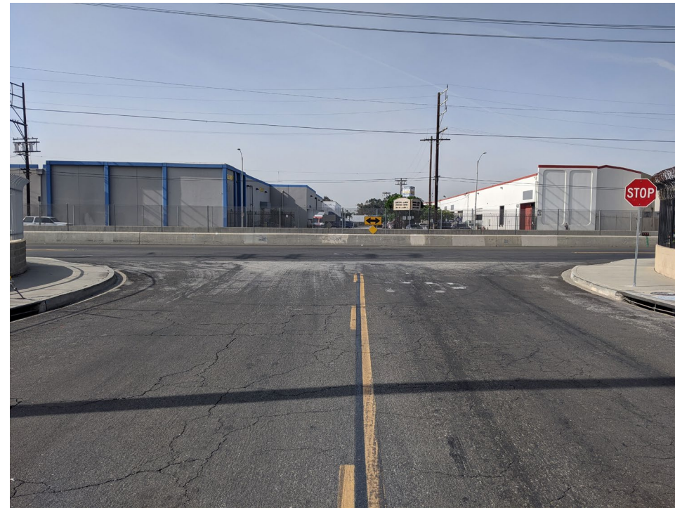
Intersections along Alameda East are designed to support access/ ingress by larger freight vehicles featuring wider turning radii.
